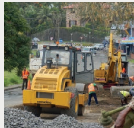
Left: Knolly Street (Suva) – good practice; laying new pipes to minimise the need to dig up the newly rehabilitated road. Photo: Fiji Roads Authority.
