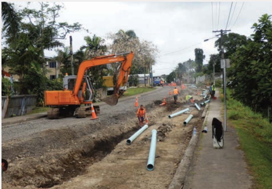
Left: Knolly Street (Suva) – good practice; laying new pipes to minimise the need to dig up the newly rehabilitated road. Photo: Fiji Roads Authority.
